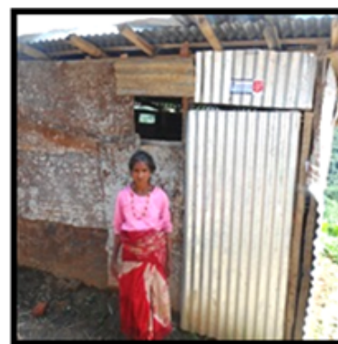
Figure 1 Earthquake Victim, Jagat kumar from Dadagaun Jitpur in front of her temporary shelter supported by VIN and SA
