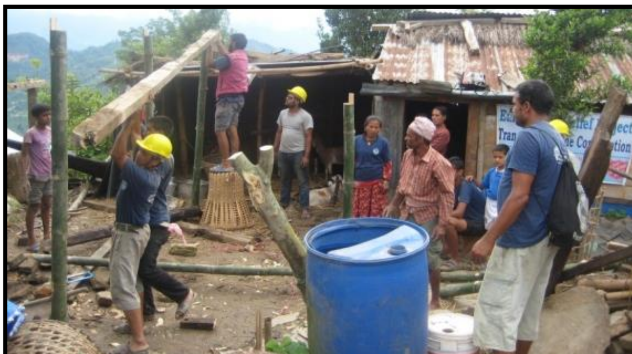
Figure 23 Transitional Homes under construction
