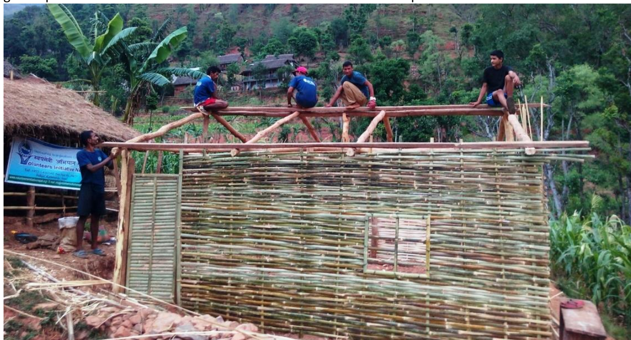
Figure 13 Transitional Homes under construction
