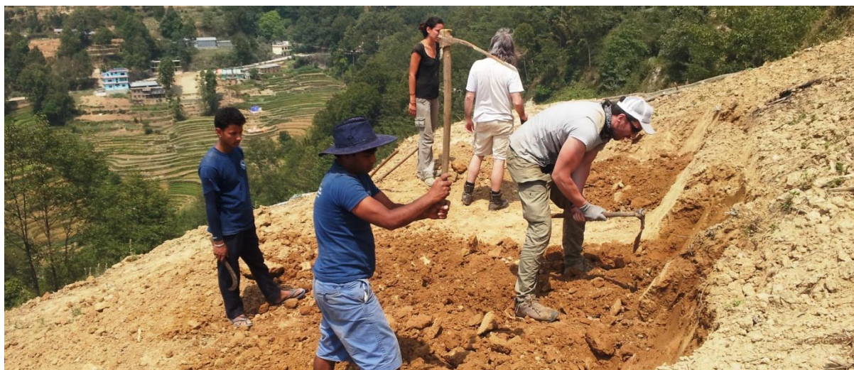
Figure 9 VIN's staff and volunteers worked to prepare land for Transitional Homes
